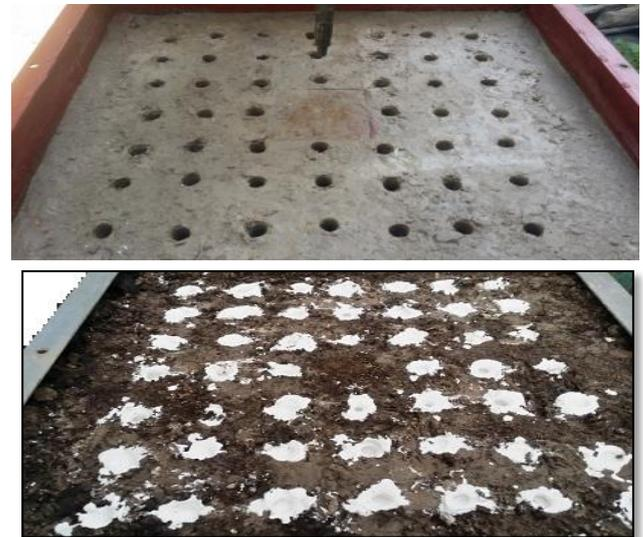
Figure 1: Lime pile installation process.
